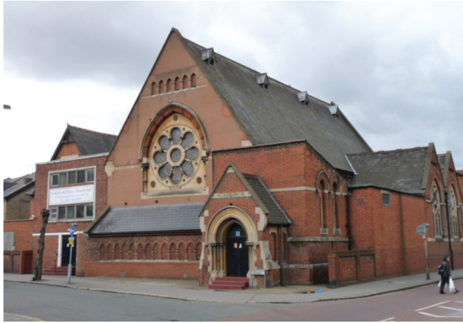
Croydon Masonic Hall Oakfield Road
