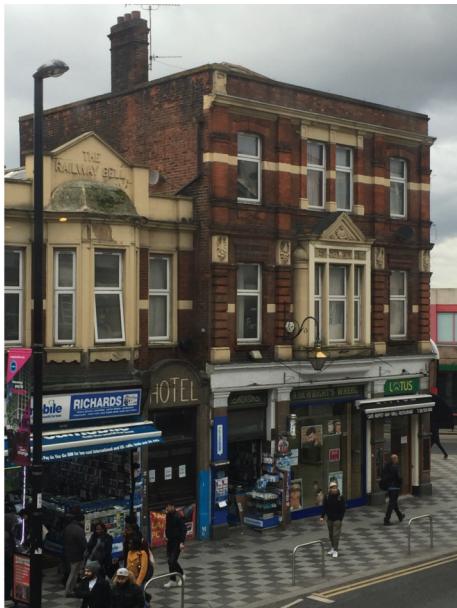
Railway Bell, West Croydon
